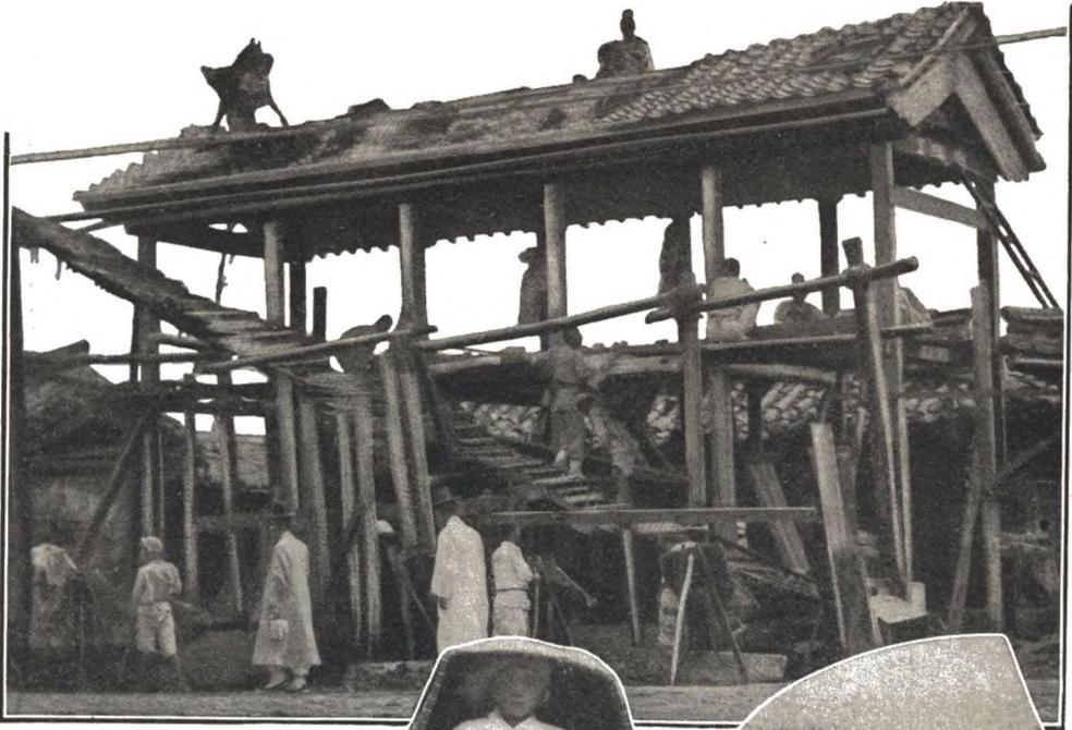
Korean methods of building—The roof is put on first of all, and the upper storeys are reached by a sloping gangway.
